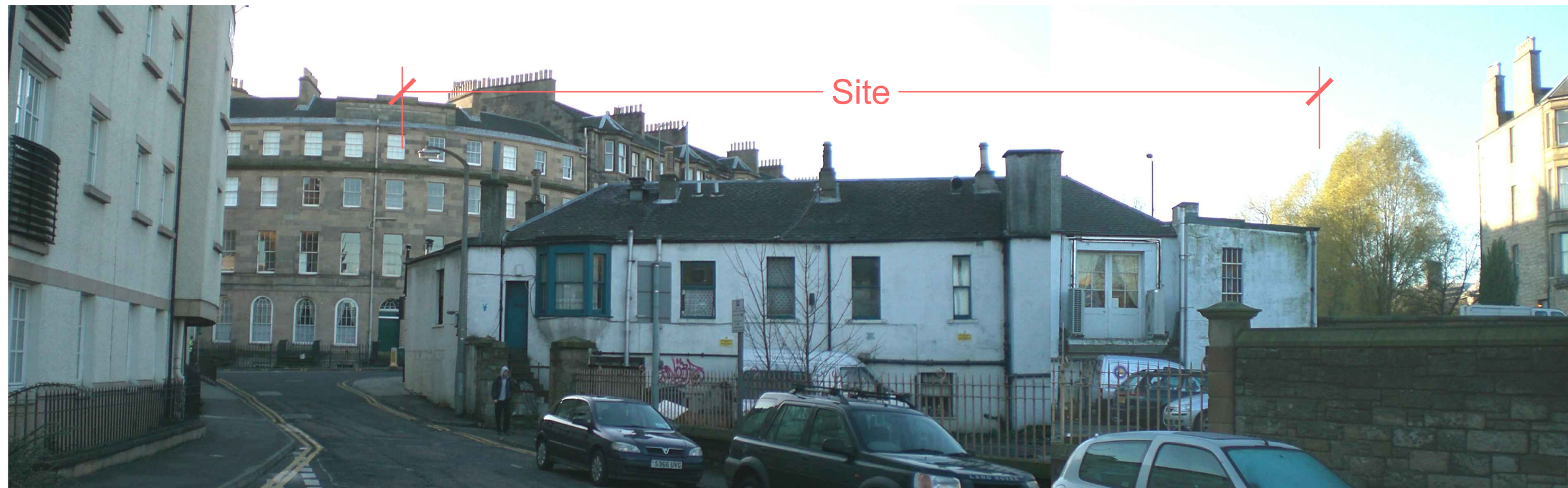
VIEW OF REAR OF BUILDING FROM NORTH EAST (Photo taken from Warriston Road)
