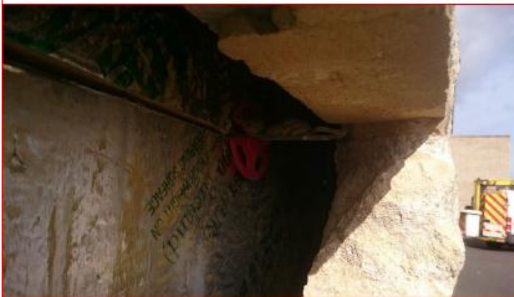
Photo 0187 Location 61B – Embedment 24mm
