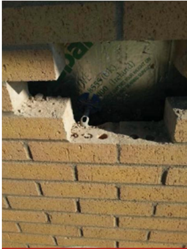
Photo 15.23.45 Location 40 – 35mm embedded
