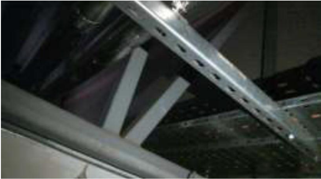
Image 21: Example of a breach of fire compartmentation from fire-stopping survey of Oxfangs School, dated 22 nd August 2016: "there is no plasterboard above the fire door, therefore creating a large breach in the compartment. the area is not fire stopped and a breach exists."
