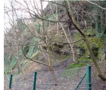
Mudstone exposure underneath the Dean Bridge (CEC)
