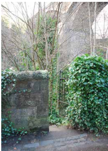
Gate to Miller Row riverside space
