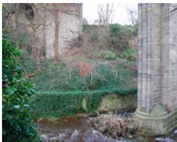
Retaining wall under Dean bridge. Most of the riverbanks have retaining structures along them, not benefiting from design by Telford but similarly affected by ivy
