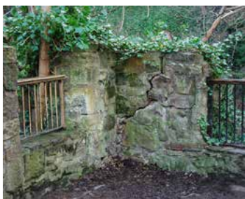
Cracked walls, ivy, rotten handrails and rusty railings at Lindsay's mill space
