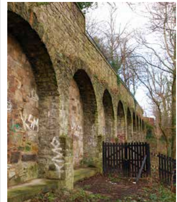
Retaining wall at top of India Street bank and below Doune Terrace Gardens
