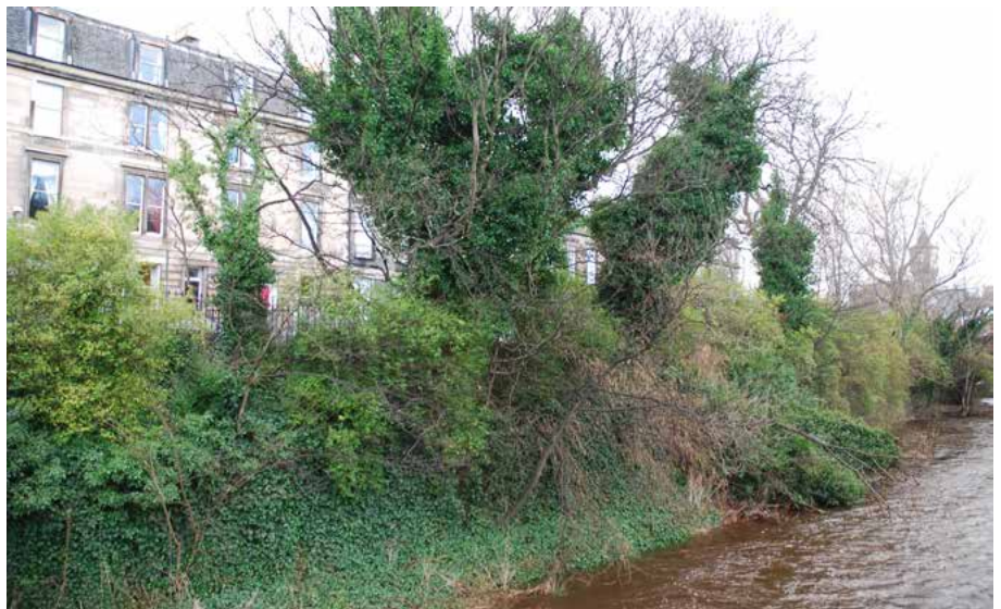
Riverbank at Upper Dean Terrace
