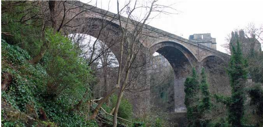
Dean bridge from Belgrave Crescent Gardens
