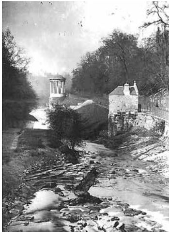
Prof Chrystal, Dean valley with the two wells and walkway, c1900-10 (RCAHMS)
