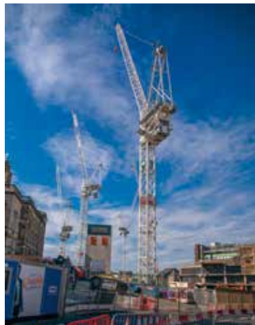
Work continues at Edinburgh St James | Photo Credit: Martin P McAdam
